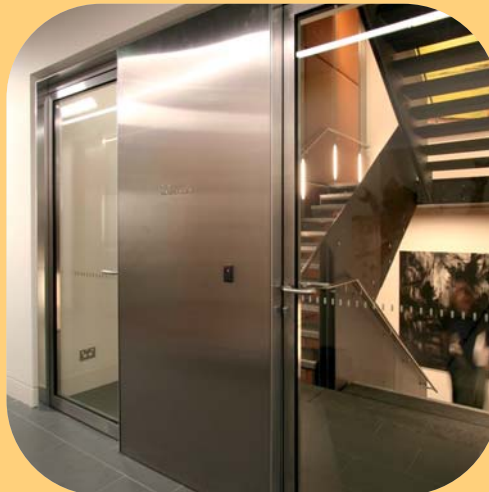
Insulated stainless-steel/glass fire doors with Pilkington Pyrostop ® – office building, Sydney, (Aust).
